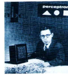
Fig. 1.4. • Frank Rosenblatt (the inventor of the perceptron and designer of the 1 Perceptron neurocomputer) with the 400 pixel (20 × 20) Mark I Perceptron sensor. Photo courtesy of Arvin Calspan Advanced Technology Center.
